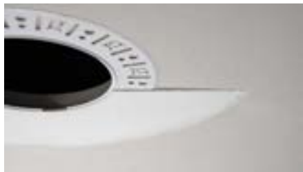
Partially finished mud ring, showing cross-section detail.
